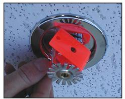
Figure 1: Sprinkler shield being removed from a pendent sprinkler.
