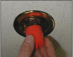
Figure 2: Sprinkler cap being removed from a pendent sprinkler.
